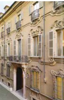
■ Palazzo Rota Pisoni (18th century) Façade on via Sant'Eufemia
