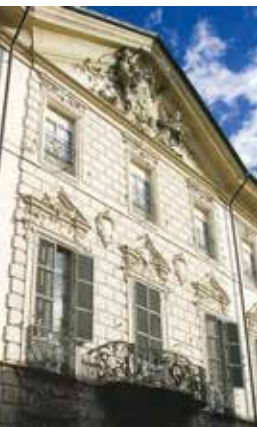
■ Palazzo Costa (end 17th century) Façade
