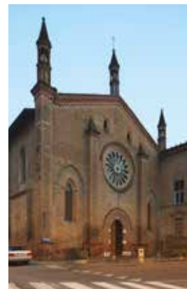
■ Saint Anna's Church (from 1334) Façade
