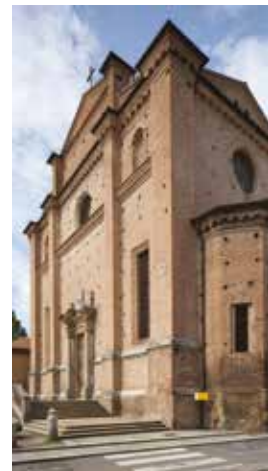
■ Saint Sepolcro's Church (early 16th century) Façade
