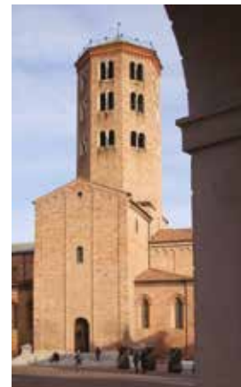
■ Saint Antonino's Church Bells tower (11th century)
