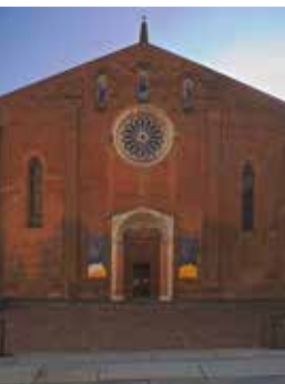
■ Church of Saint Giovanni in Canale (1121-1270) Façade
